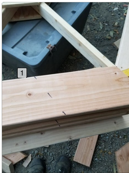
1. mark 20 1/2" from the bottom, parallel to the cut
