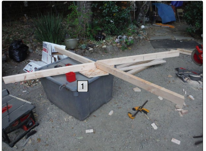
1. place the assembly on a raised platform and attach screws from underneath to save time
